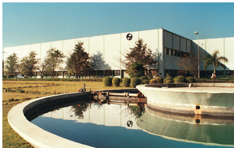
Switchgear Factory, Ahmednagar
