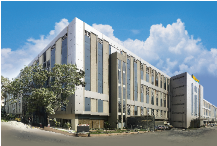
Switchgear Factory, Mumbai
